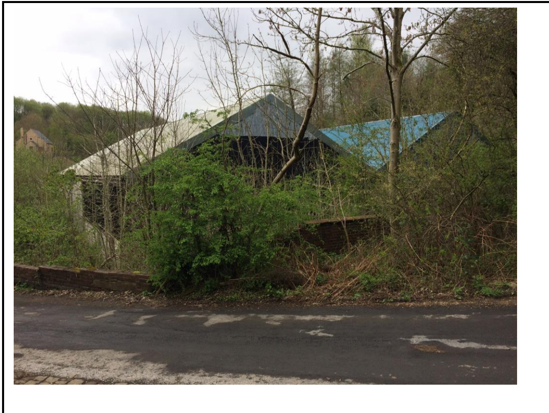
Photo 4 – view looking westwards from the eastern boundary of the site
