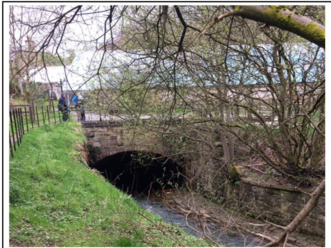
Photo 6 – view towards the southern edge of the site, with the bridge over the River Medway on Mill Brow in the foreground.
